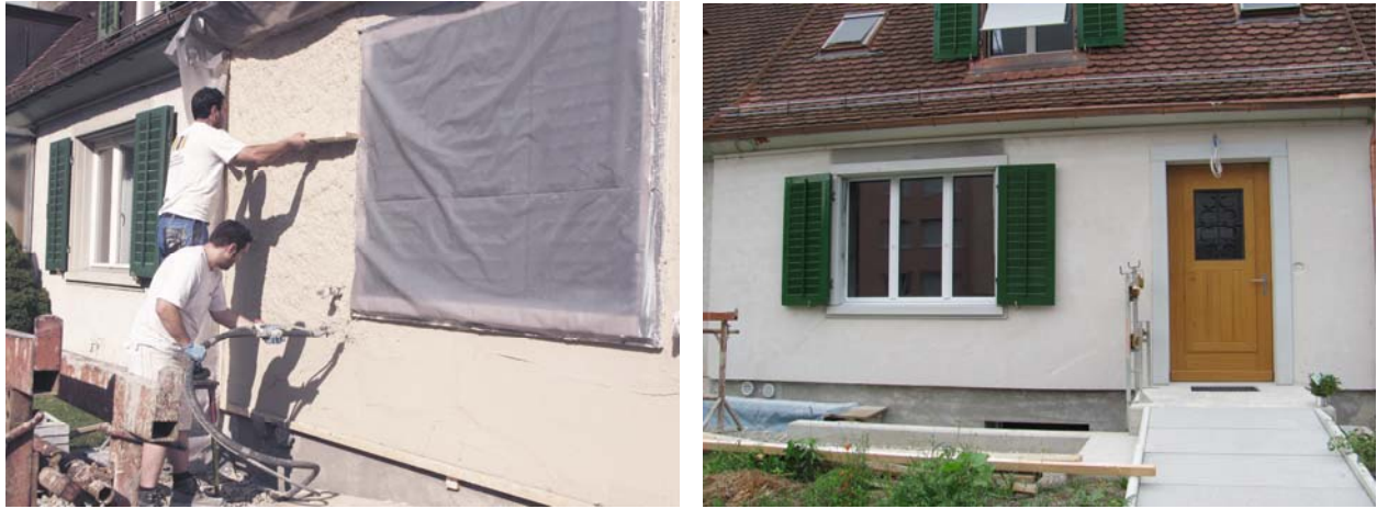
Figure 18: Renovation of an old row house in Winterthur: spraying and equalizing of aerogel render (left), aerogel render before application of finishing render
