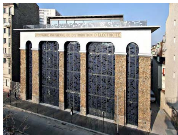
Figure 29: Good solar integration in an historical context is often a challenging task and creates extra costs: Substation of Electricité de France (EDF) built in 1929 and converted into an "Industrial Hotel" for start-up companies – 123 kWp [7]
