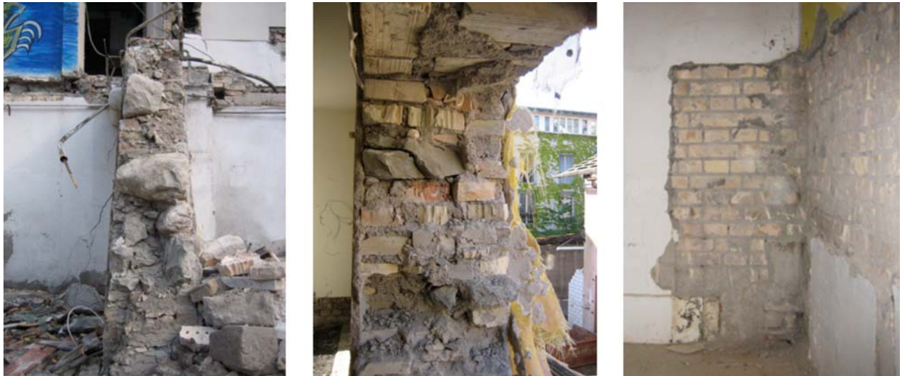
Figure 4: Typical wall constructions: natural stone wall (Seefeldstrasse), mixed masonry wall (Feldegstrasse), brick wall (Kernstrasse)
