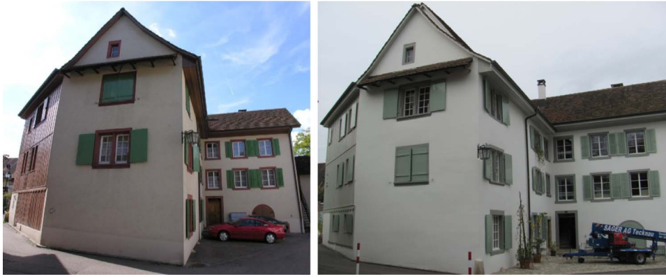
Fig. 1. Eastern façade of the building before retrofit with the portland cement rendering (left) and after retrofit with the new aerogel based rendering (right).
