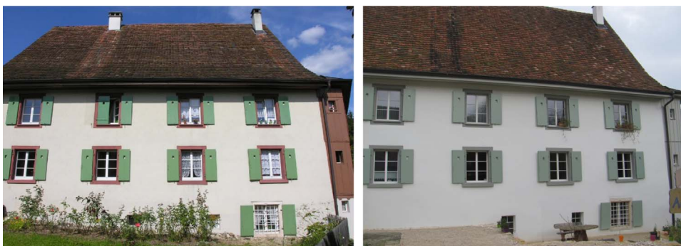
Fig. 2. Southern façade of the building before retrofit with the portland cement rendering (left) and after retrofit with the new aerogel based rendering (right).
