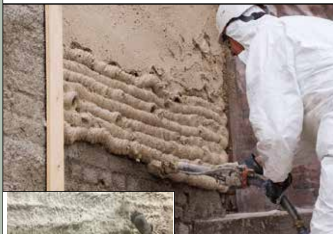
Figure 22- Image one: The clean surface, ready for application of the undercoat layer. Second image: The surface with undercoat layer. When the undercoat is dry, a layer of Fixit222 can be applied (Source: Bolligbygg).
