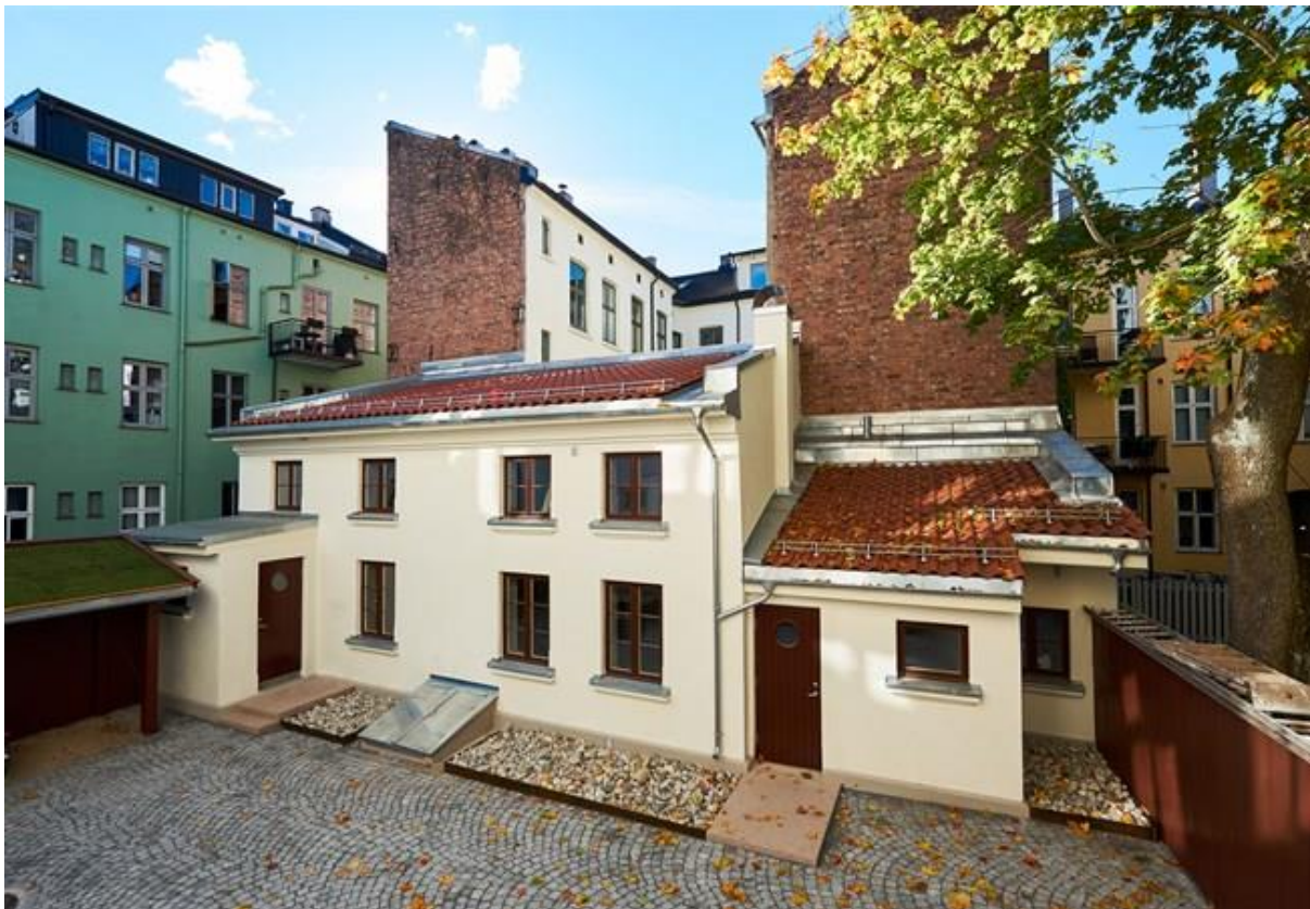
Figure 18: The northeast façade of BG12B-C after refurbishing. Photo: Eivind Røhne/FutureBuilt.
