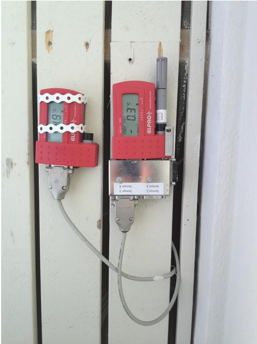
Figure 35- Two Elprolog logger units mounted under the cornice.
