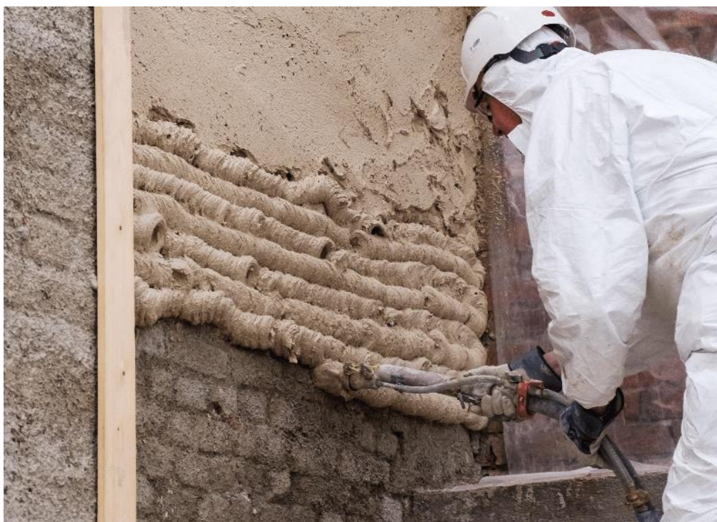
Figure 23- A worker applying Fixit222 with a spray gun ((Source: Boligbygg).
