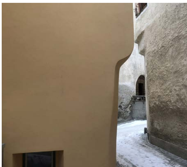
Here the facade created with Aerogel insulating render is telling a story that is still understandable in its context.
