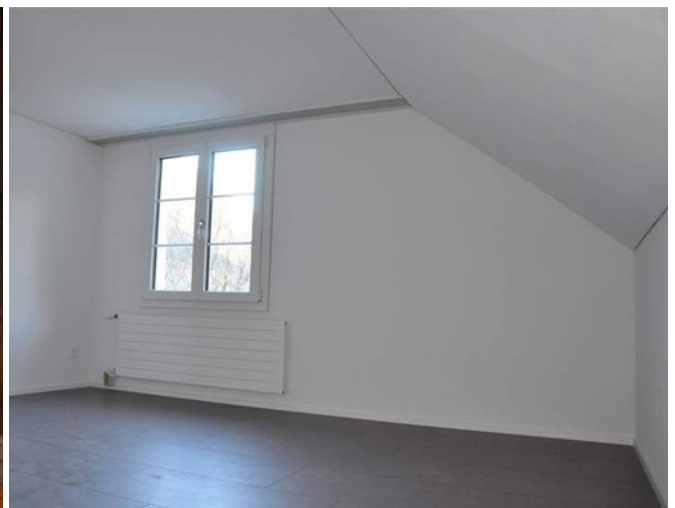
Indoor insulation using facing formwork
