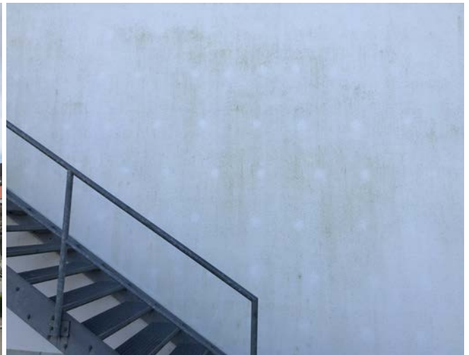
10-year-old facade of thermally insulating render
