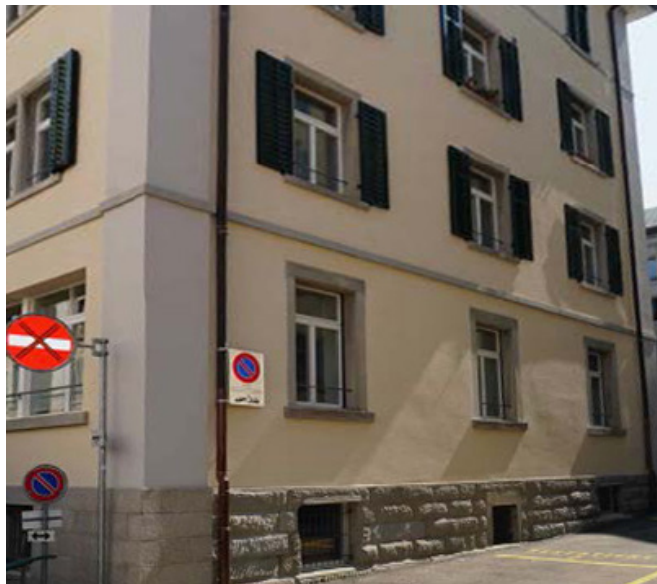
Facade of Aerogel insulating render. The insulation is not visible.
