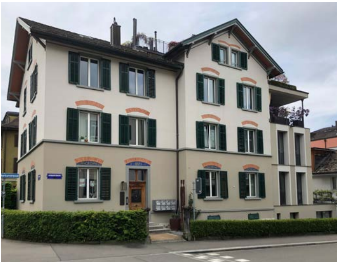
10-year-old Aerogel facade given no maintenance
