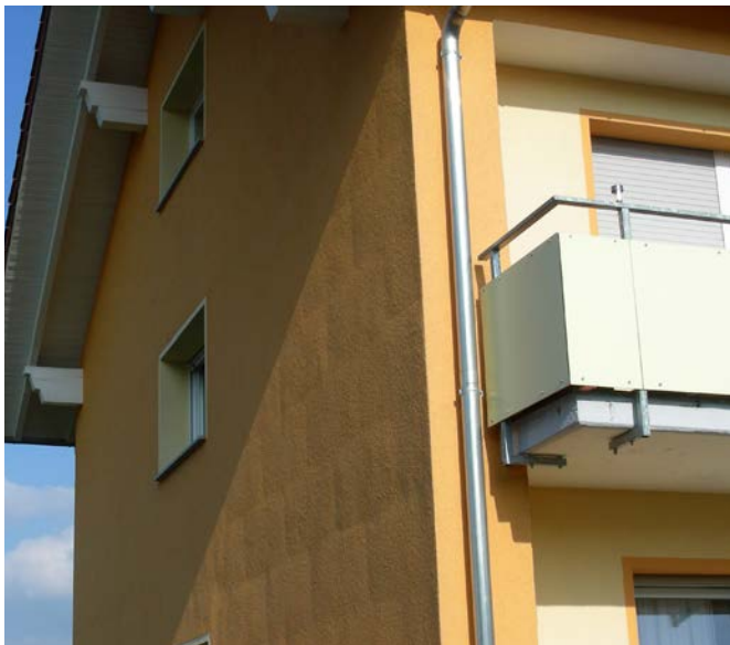
Facade of insulating panels illuminated in angled light. The outline of individual panels is visible under the surface but in accordance with SIA 243 «Rendered exterior thermal insulation» must be accepted as such.
